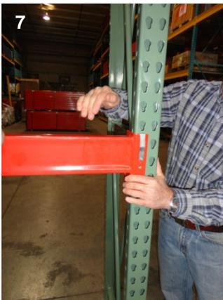
While steadying the Upright Truss with the Beam connected and locked in place, raise another Truss and connect the Beam as previously outlined, and as shown in photographs 7 and 8. Continue working in one direction setting up rack bays. Do not set up bays from two ends working toward a center.
