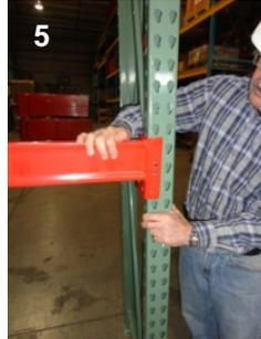
Seat the Beam, as shown in photographs 4 and 5, by engaging the studs in the beam end plate into the keyholes of the column. The beam is correctly seated when the H001 Spring Clip slides into the top of the end plate and can then be locked in place by inserting the stud into the hole in the end plate and column as show in photograph 6.
